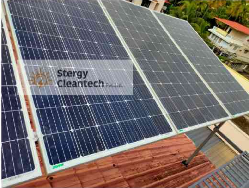
5 KW PROJECT SANAL KUMAR THRISSUR
